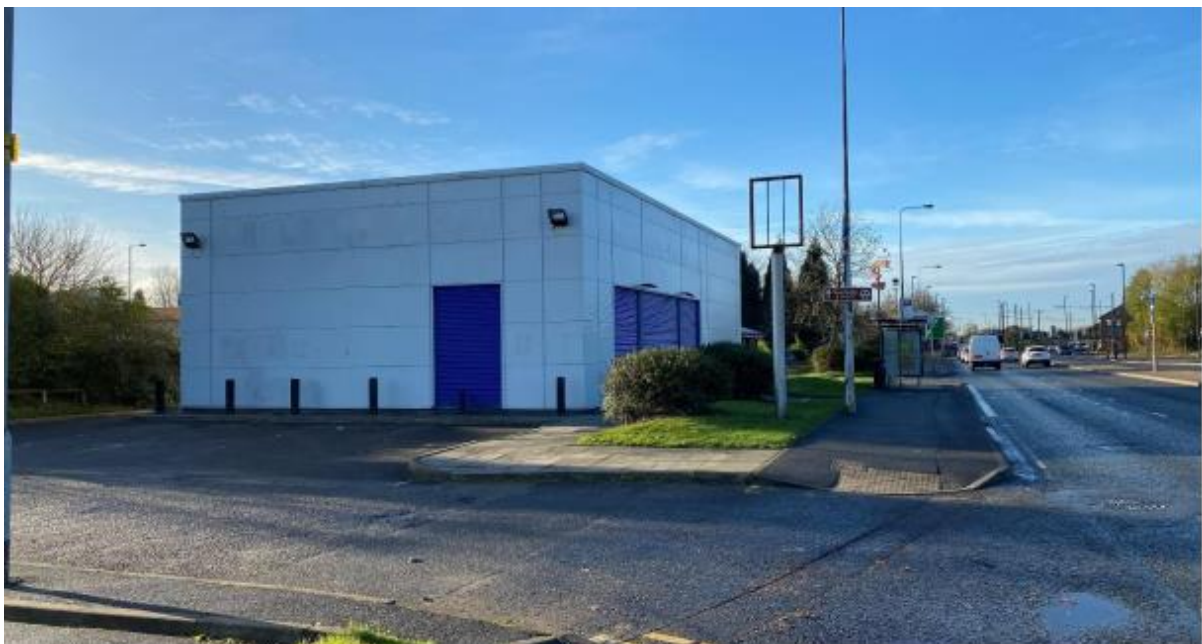
Photo 5: Vacant former Carphone Warehouse building
